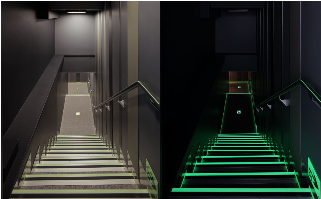
Stairwell with Photoluminescent system in natural light
